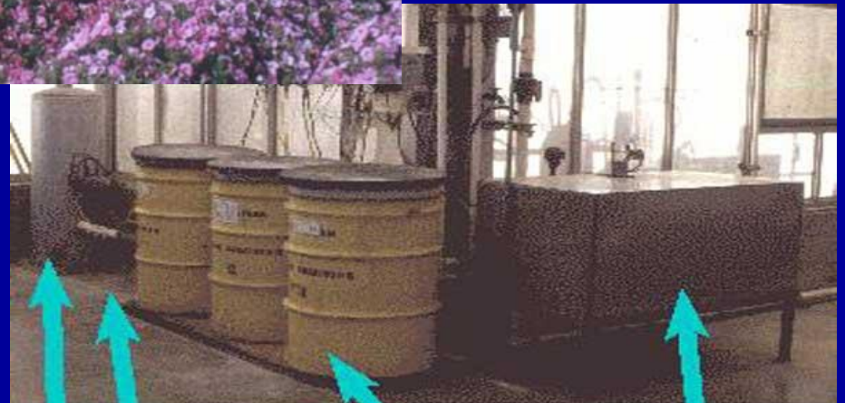
Injectors Mixing tank Stock solutions Holding tank
